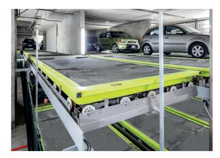
In 2015, *Lödige Industries* installed the first automated parking system in Ottawa. It provides parking for 47 cars in *The Eddy* building, a six-storey condo tower. The main challenge of this building was an unconventional footprint requiring a customised parking solution. The *5BY2* pallet-based technology from *Lödige Industries* enabled a maximum of parking slots for this unique building.
